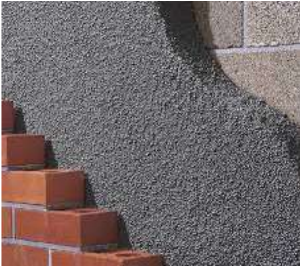
Section of Building showing Bead Insulation
